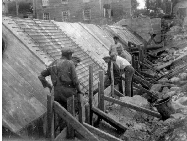
Setting rebar, from an album of the estate of Edith Onderdonk estate, © Durham Historical Association.
