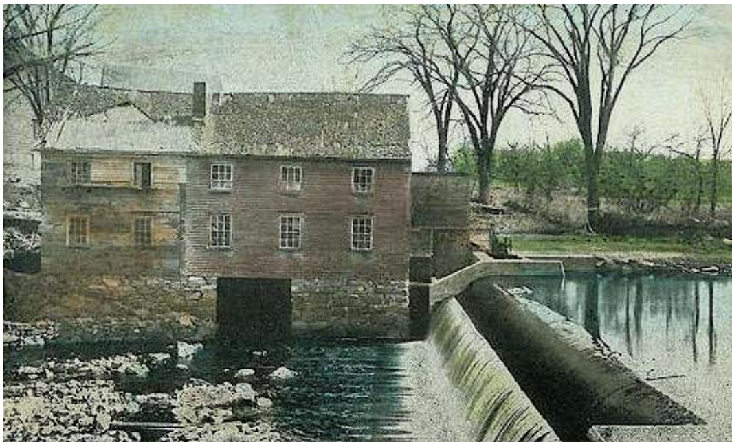
Jenkins Mill and Mill Pond Dam, from 1908 postcard.
